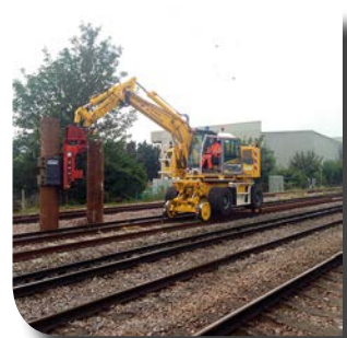
Installation of electrical overhead lines, UK
