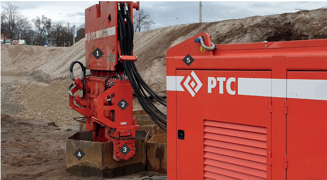
1 Yoke / Extraction box | 2 Vibrator gearbox | 3 Clamping head | 4 Profiles | 5 Power pack
